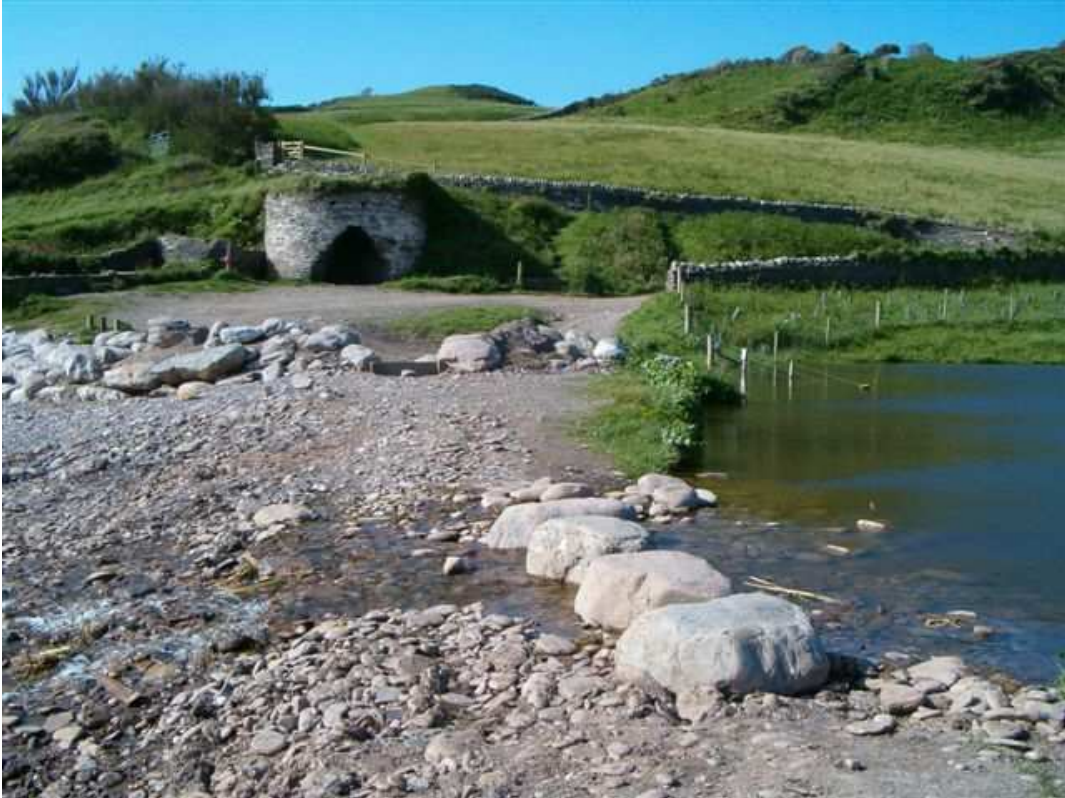
Coast Path prior to breach
